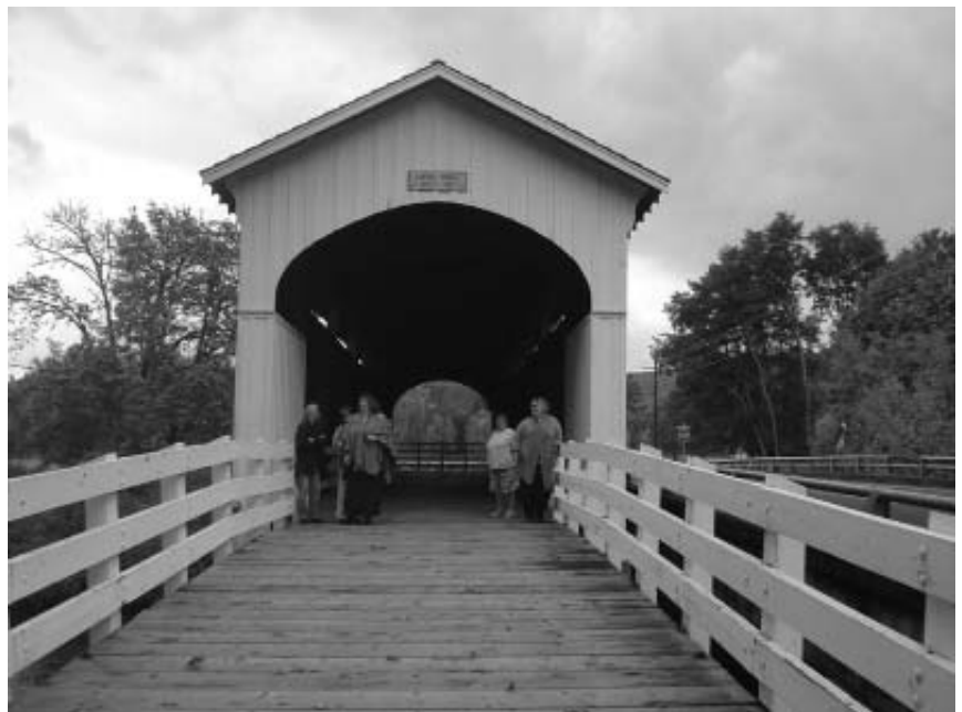
The Currin Covered Bridge
